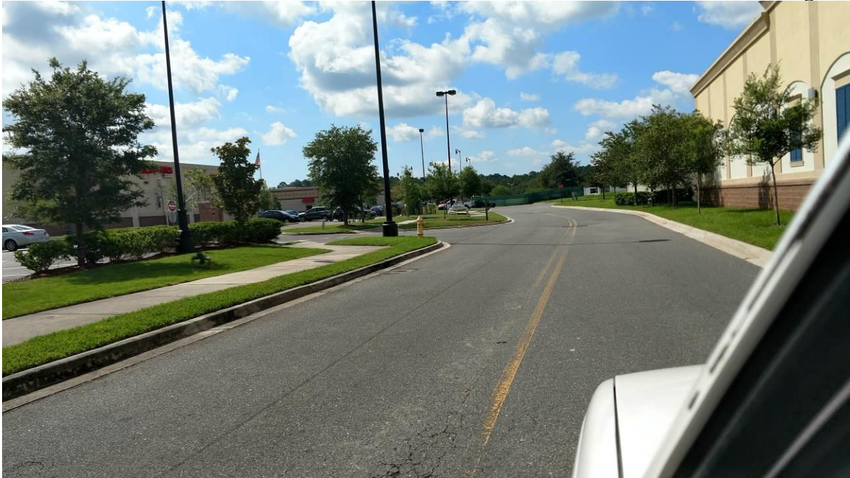
Improved Nautica Drive to the west of unimproved section
