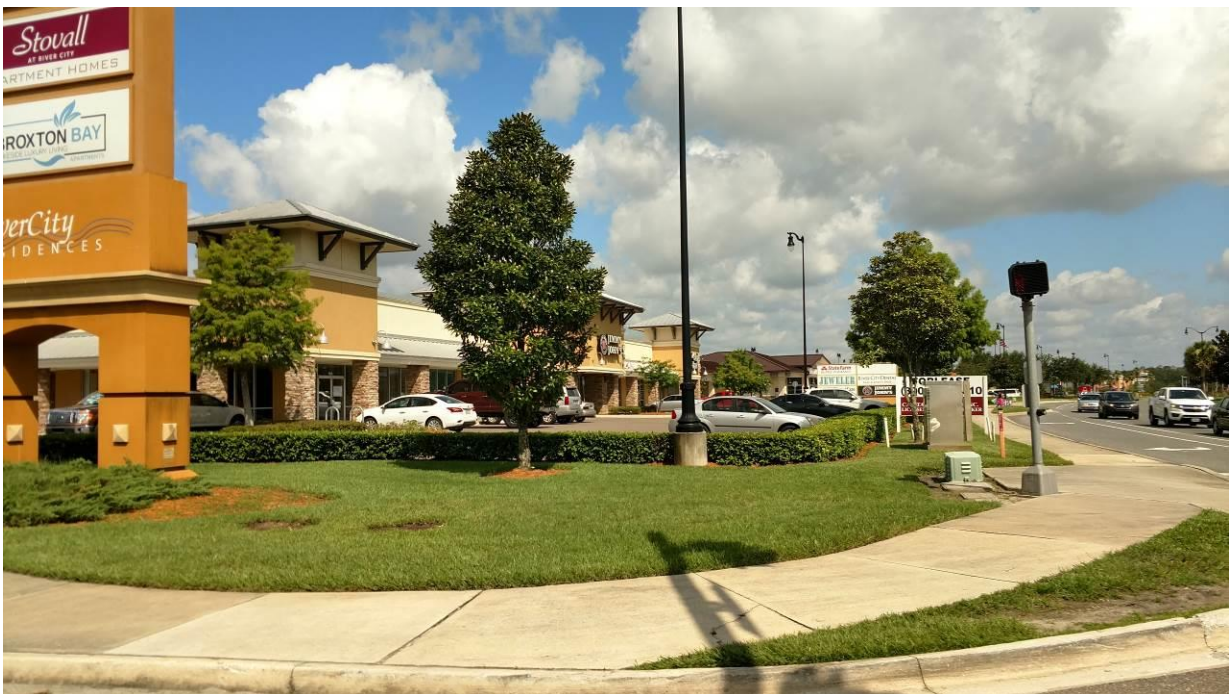
Commercial to the north of Nautica Drive right of way Source: Staff, Planning and Development Department Date: 07.07.2017
