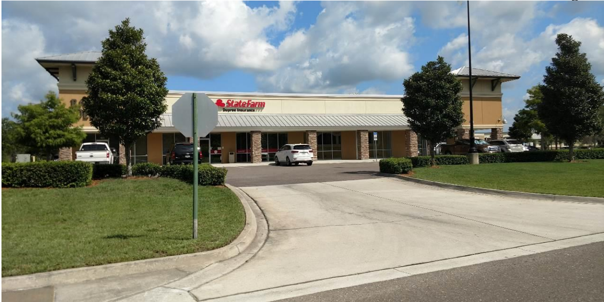
Commercial to the north of Nautica Drive right of way Source: Staff, Planning and Development Department Date: 07.07.2017
