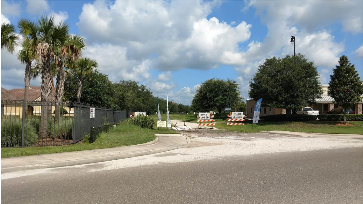
Unimproved Nautica Drive Right of Way Source: Staff, Planning and Development Department Date: 07.07.2017
